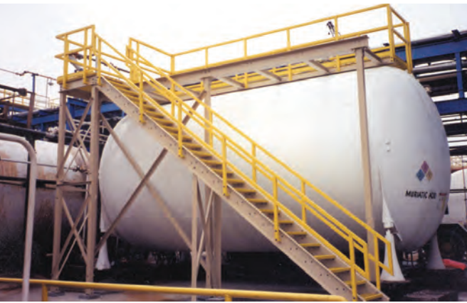
SAFRAIL™ system in a chemical plant.
